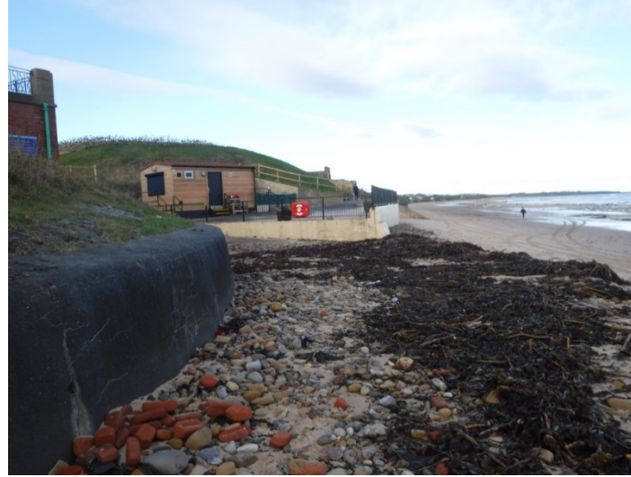
Plate 2 – Survey photograph 1aNTDC04_20151126_N3
